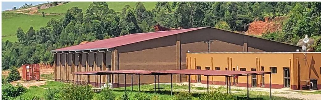
[Reconstructed Chapel Building (250115)]
